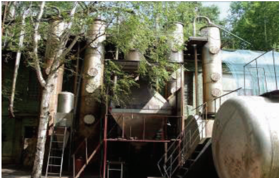
HRCM industrial production
