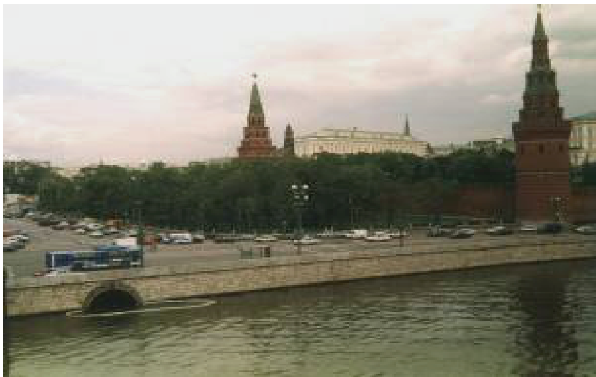
HRCM boom protection on Moskva River
